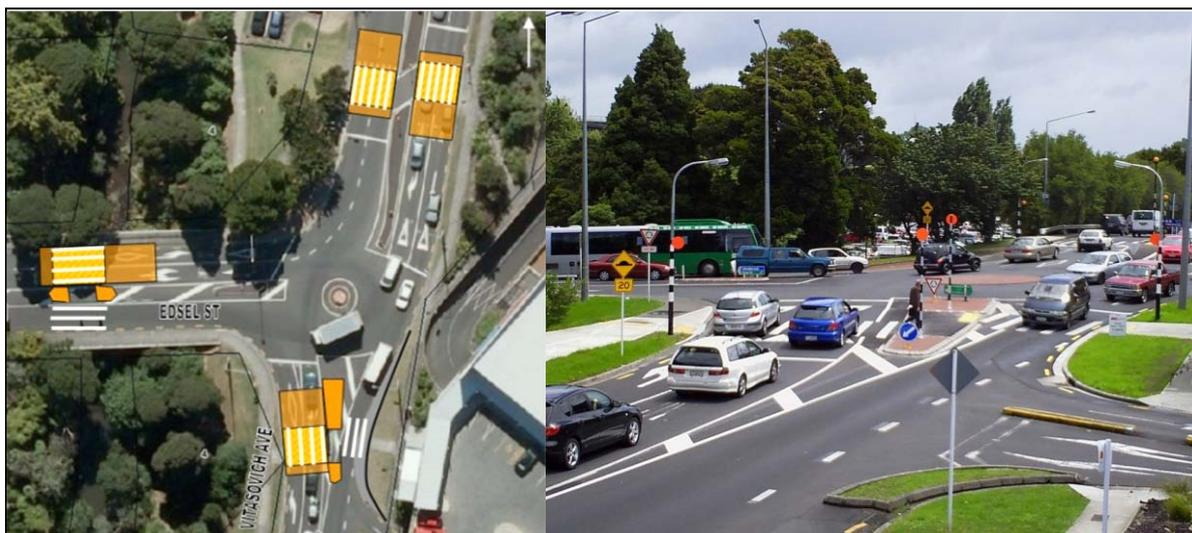
**Figure 3: 'Directional' platforms were installed in 2010 at the Vitasovich Ave / Edsel St roundabout in Auckland (although not all platforms were constructed to the specified heights).**
