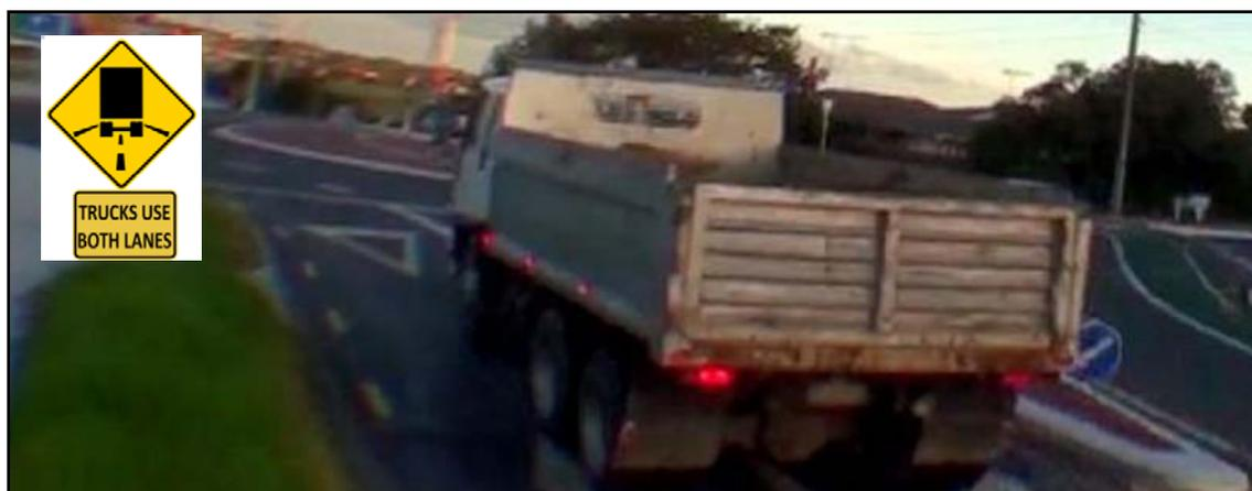
**Figure 1: Truck straddling the two narrow lanes on approach to a C-Roundabout. Although fairly intuitive to drivers, advance warning signs are considered desirable with an example used shown inset.**
