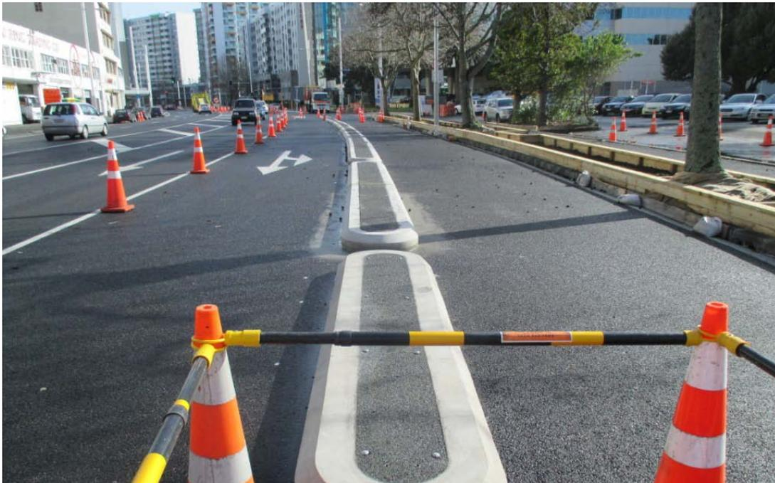
**Figure 8 – Raised Kerb Separator (Under Construction)**
